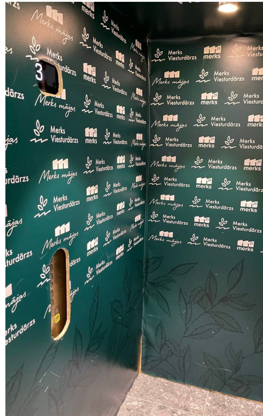
Elevator branding during construction.
