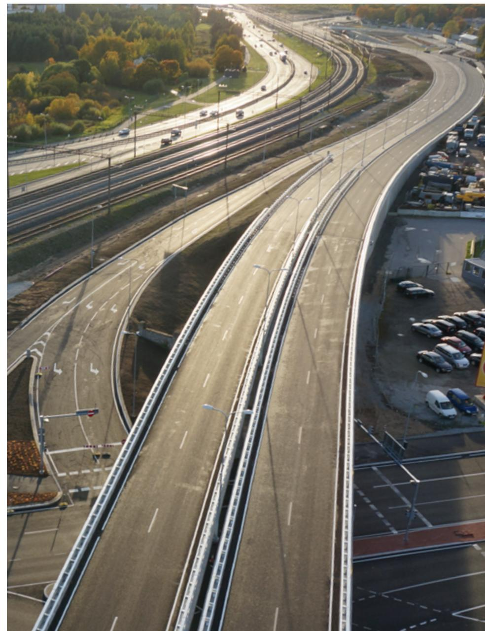
AT THE CONSTRUCTION OF ÜLEMISTE TRAFFIC JUNCTION, 8.7 KM OF CARRIAGEWAY AND 7 KM OF NON-MOTORISED CYCLE AND PEDESTRIAN TRACKS WERE BUILT AND 155,000 SQUARE METRES PAVED WITH ASPHALT.
