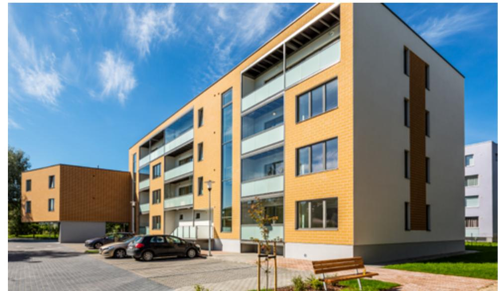
THE RÄÄGU 9 APARTMENT BUILDING IN TALLINN HAS A CATEGORY A ENERGY LABEL. COMPARED TO APARTMENT BUILDINGS COMPLETED IN THE PAST, THIS ONE HAS THICKER INSULATION IN THE EXTERIOR WALLS AND ROOF, ALSO TRIPLE PANE WINDOWS.
