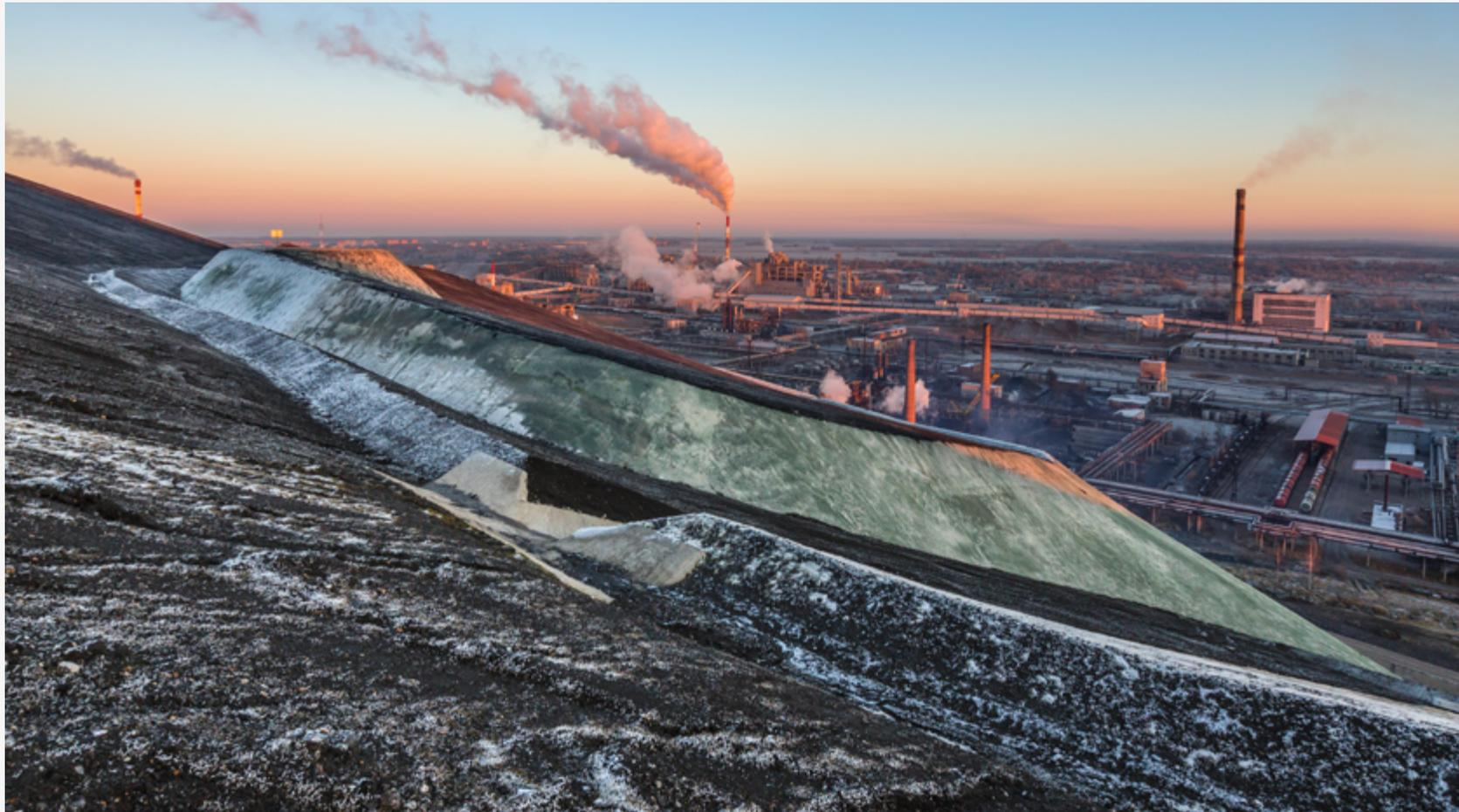
WITHIN FIVE YEARS OF WORKS AT CLOSING THE KOHTLA-JÄRVE INDUSTRIAL WASTE AND SEMI-COKE DUMP IN NORTH-EASTERN ESTONIA, A HILL OF MINE WASTE AMOUNTING TO 6 MILLION M<sup>3</sup> WAS RELOCATED, 84 HECTARES WERE REPLANTED, A RAINWATER COLLECTION SYSTEM MORE THAN 8 KM LONG WAS INSTALLED, AND 2.5 HECTARE LAKES CONTAINING LIQUID OIL SHALE MINING RESIDUES WERE CLOSED.
